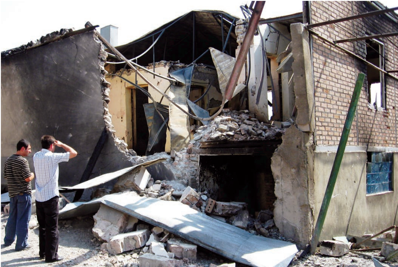
The IRC surveys homes destroyed by recent bombings in Ruisi, one of the villages surrounding the town of Gori, in Georgia.
