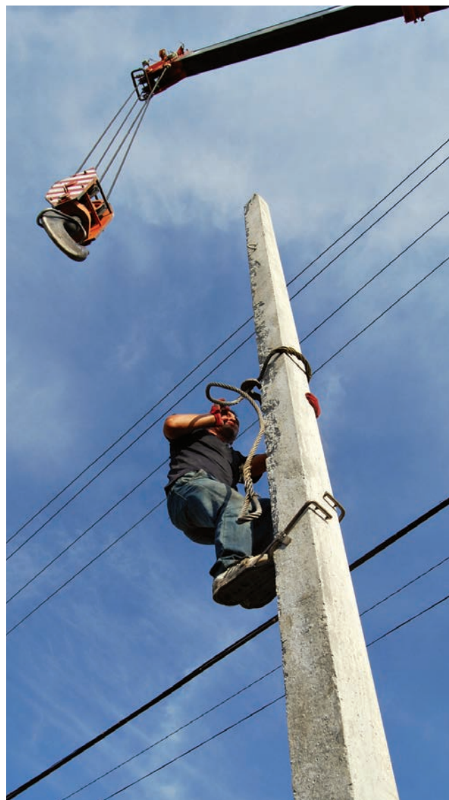
Here in a neighbourhood in Osh, Kyrgyzstan, the IRC is providing more than a dozen new power poles. Made of steel and concrete, the posts should last decades.
